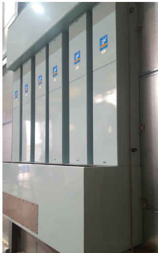
Installed MPE HEMP filters with custom fabricated mountings
