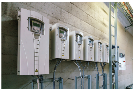
Array of variable frequency drives in situ
