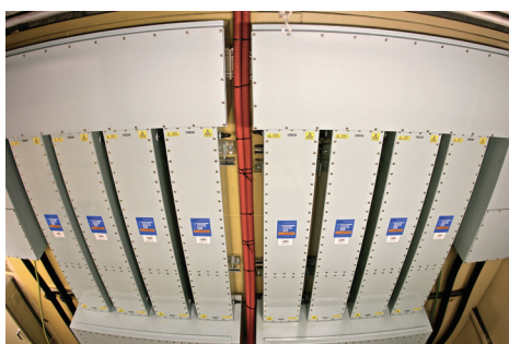
Array of MPE HEMP filters in service at RAF Fylingdales in North Yorkshire
