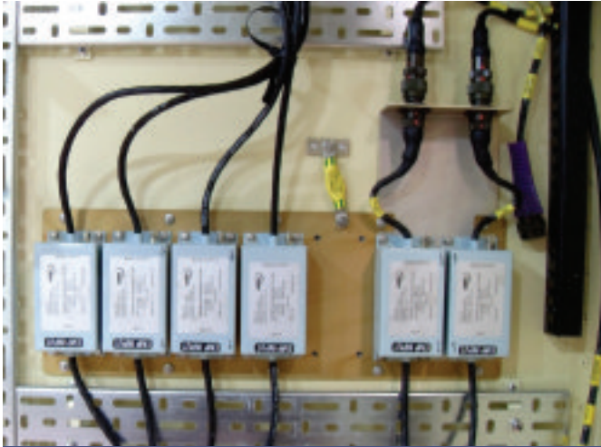
TEMPEST EMI equipment filters as installed in a battlefield enclosure.
