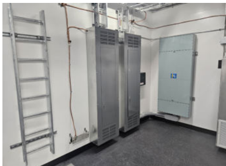
Inside of the Armag modular A.R.C. vault shelter with its MPE Extended Performance TEMPEST power line filter installed on the back wall
