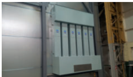
A suite of very high current (VHC) power line filters of various current ratings, including custom 2500V DC 2000A units complete with end enclosures, have been integrated into a major UK test chamber installation. Those MPE DC filter units, pictured here in situ, measure 3m high by 2m wide and weigh two tonnes.
