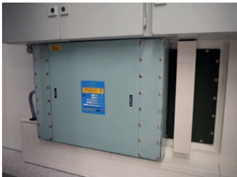
Close-up of the 32A MPE high-performance power line EMC filter in situ
