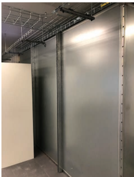
External views of the RF chamber designed, manufactured and installed by NTD Shielding Services for BBC Research & Development's South Laboratory in West London
