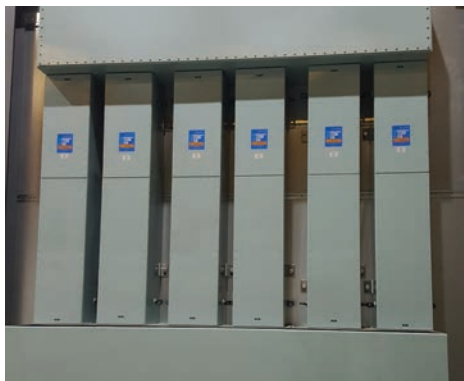
Installed high-current MPE filters provide essential EMC protection for incoming power lines
