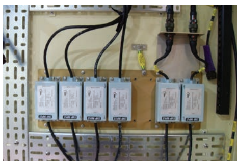
An array of MPE TEMPEST EMI filters in a tactical shelter
