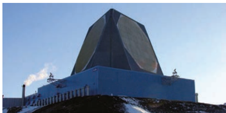
MPE has supplied a suite of Mil-Std-188-125 HEMP filters for the Ballistic Missile Early Warning System at Thule Air Base on the north-west coast of Greenland, the northernmost base of the US Air Force
