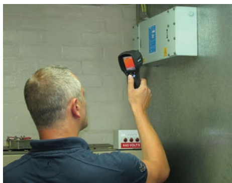
Thermal imaging is used for checking an installed power line filter
