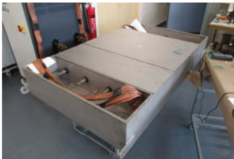
MPE filter during current overload testing at MPE, Liverpool
