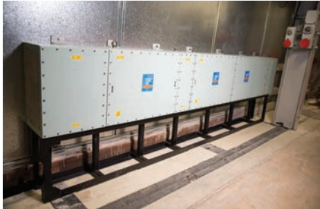
MPE 800A 1500V DC filters mounted onto the anechoic chamber at Horiba MIRA, Nuneaton
