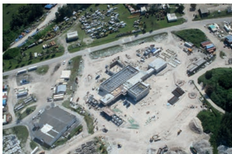
Current construction of the sensor site on Kwajalein Atoll
