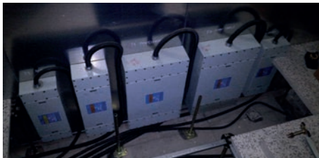
The MPE filters in situ at JIAT
