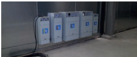
MPE filters during their installation by Eretec at JIAT
