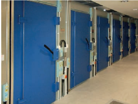
MPE powerline filters mechanically fitted and electrically connected to the doors of an MVG shielded room
