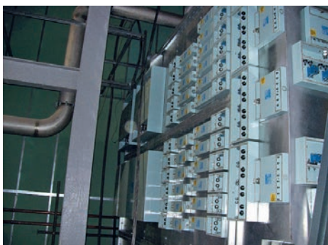
MPE powerline filters mechanically fitted and awaiting electrical connection on the outside of an MVG test chamber
