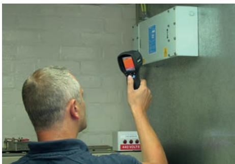
Thermal image checking of filter
